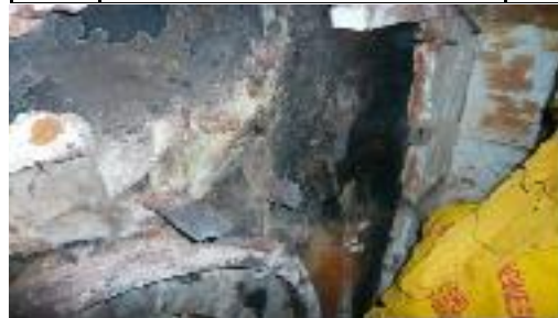
REFRACTORY WORK - In the removing process of damaged Fire brick at Boiler
