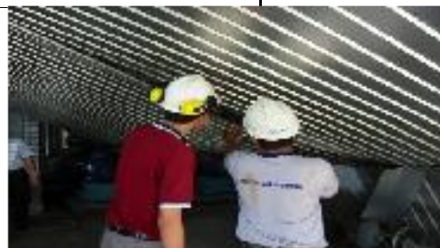
ALIGNMENT WORK- Alignment seal of Diverter Damper at TNB Generation of Klang
