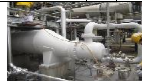
PROJECT CUI - Removal, replace of insulation and cladding and finished with industrial painting for the corroded equipment at Titan Group
