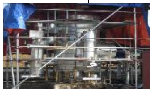
SCAFFOLDING WORK - Erection scaffolding shelter with Canvas
