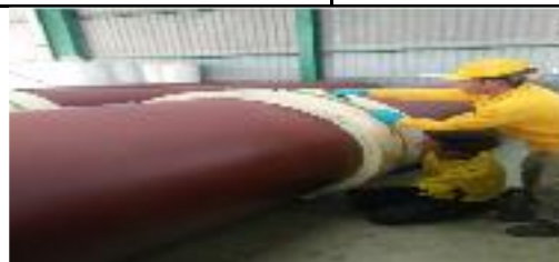
COLD INSULATION WORK- PIR Installation Insulation for LNG Piping at Pengerang Dialog Warehouse, Johor
