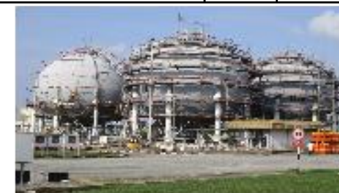
PROJECT BHP 2015 - Erection and Dismantle of scaffolding work for 14 nos tanks and complete with industrial tanks at BHP Johor Port
