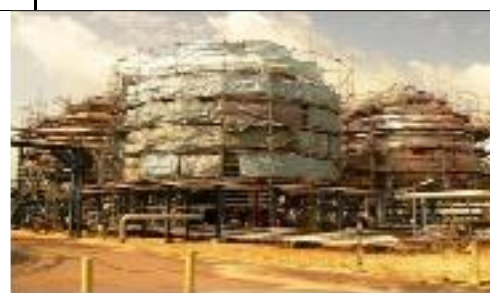
TITAN - TK5110A,B,C,D&E Cold Insulation Cladding Replace Work (2012)
