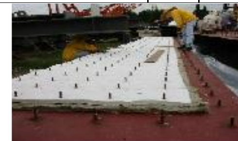
CERAMIC INSULATION - Installation of Kaowool / Ceramic for Furnace at EESB PD Power Station
