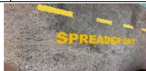
PAINTING LABELLING WORK - Labelling work with Termoplastics for ASIAFLEX Plant at Tg Langsat
