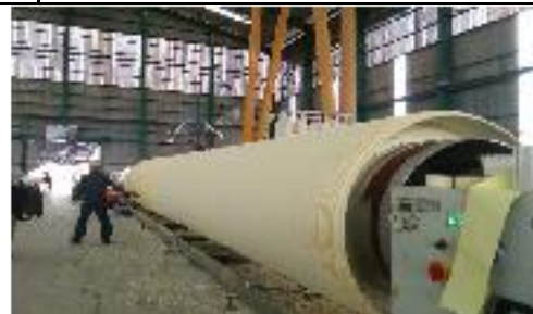
COLD INSULATION WORK- PIR Installation Insulation for LNG Piping at Pengerang Dialog Warehouse, Johor
