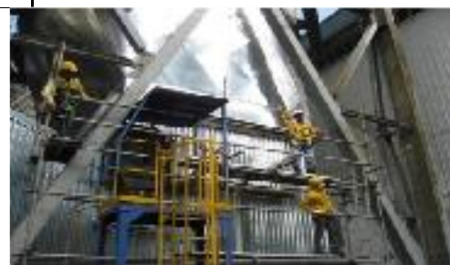
SCAFFOLDING & INSULATION WORK - Removal and Renew of Cladding and Insulation at TNB Generation
