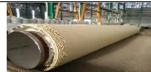
FIBERGLASS WORK - Applying of Fiberglass onto the severe damaged cable duck at PPE Titan Group
