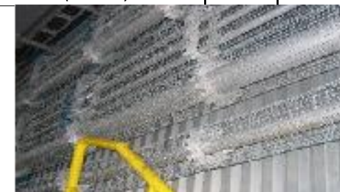
INSULATION WORK- Removal, replace of insulation and cladding and finished with wired mesh for personal protection at YTL
