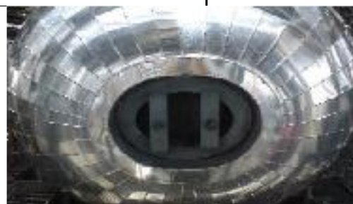
PROJECT PD2 REHABILITATION - Installation of Calcium Silicate for HP 2B Drum at Tungku Jaafar Power Station Port Dickson, Negeri Sembilan
