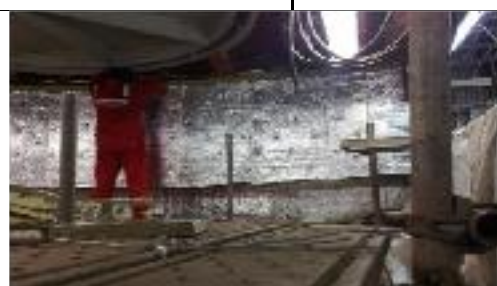
SUNBORN -Installation Insulation Of Rv & Armaflex On Decks , Stiffeners and Piping (2011)
