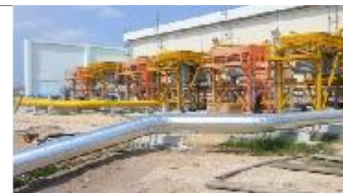
PROJECT INSULATION - Installation of Calcium Silicate for fuel gas line at EESB PD Power Station
