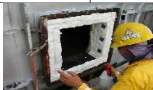
FURNACE MANHOLE INSULATION - Installation of Kaowool / Ceramic for furnace at EESB PD Power Station
