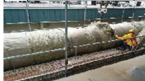
HOT INSULATION WORK - Removal and Review of Cladding and Insulation at Malakoff U-10 Boiler Outage, Johor
