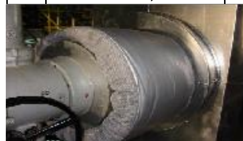
MATTRESS INSULATION - Mattress fabrication and installation for Turbine at ALSTOM POWER PLANT
