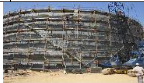
SCAFFOLDING WORK - Scaffolding for Sphere Tank for KNM Process Group
