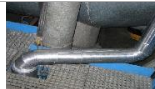
INSULATION WORK - Removal and Renew of Cladding and Insulation for YTL Cable Duct
