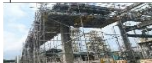
PROJECT SCAFFOLDING - Erection and Dismatle of Scaffolding Hangging and Suspension Type for TPC 1 Lotte Chemical (M)
