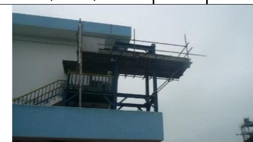
SCAFFOLDING WORK - Scaffolding Hanging Suspension Type at Lotte Chemicals Titan (M) Sdn Bhd
