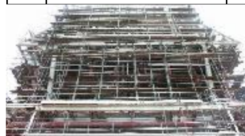
HOT INSULATION WORK - Removal and Review of Cladding and Insulation at HRSG ST 1A EESB
