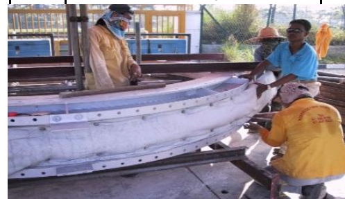
INSULATION WORK- Assembly of Expansion Joint
