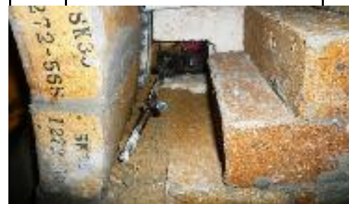
TITAN -Boiler B ( PK-3202 ) Refractory Repair Work (2009)
