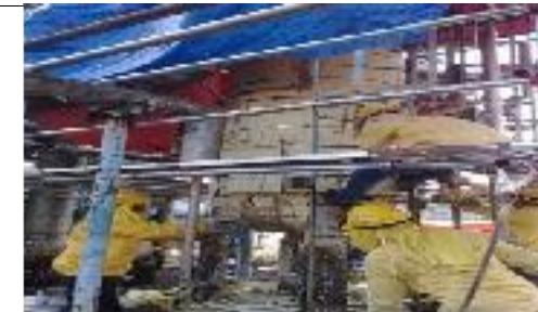
COLD INSULATION WORK - Removal & Renew of Cladding and Insulation at IDEMITSU SM tower, Pasir Gudang
