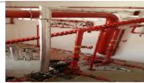
INSULATION WORK- Insulation and Cladding installation for 14 pump room
