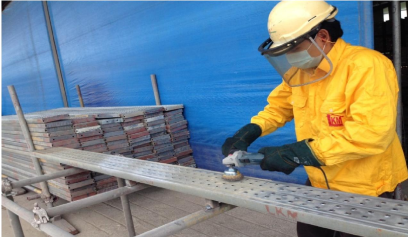
Removing of debris / scale using power tool
