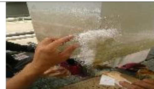
FIBERGLASS WORK - Applying of Fibreglass onto the severe damaged cable duck at PPE Titan Group
