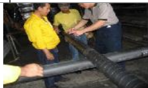
WRAPPING WORK - Removal and Renew of Denso Tape
