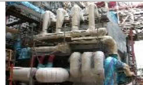
PROJECT INSULATION - Installation of Calcium Silicate for fuel gas line at EESB PD Power Station
