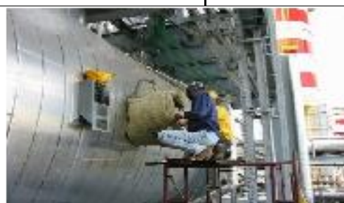
HOT INSULATION WORK - Removal and Review of Cladding and Insulation at ALSTOM POWER PLANT
