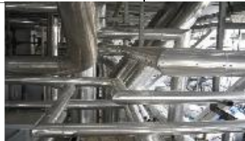
PROJECT PD2 REHABILITATION - Installation of Calcium Silicate for Injet GE Plenum at Tungku Jaafar Power Station, Port Dickson Negeri Sembilan
