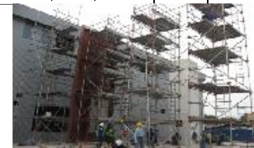
SCAFFOLDING WORK - Erection scaffolding
