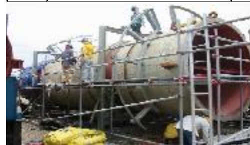
INSULATION WORK - Installation of Rockwool to the tower at Teluk Jawa Project
