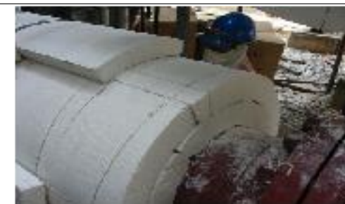
HOT INSULATION - Installation of Calcium Silicate at EESB PD Power Station GT-1
