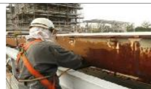
PROJECT -Corrosion Under Insulation Inspection (PIPING & VESSEL) at IDEMITSU SM(M) Pasir Gudang,JB
