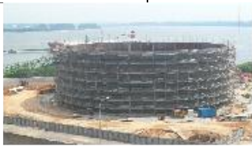
Scaffolding Work- Erection and Dismatle of Scaffolding Work for Benzene and Naptha Tank for KNM Group at Lotte Terminal 3
