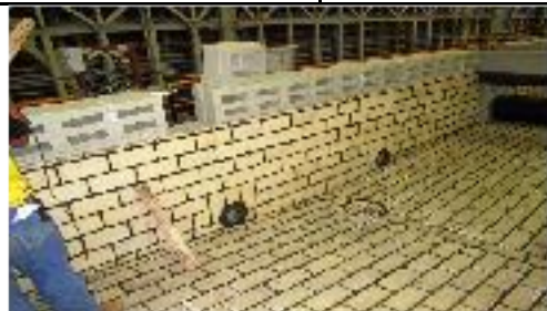
REFRACTORY WORK- Refractory work for Acid Water Tank at Bahru Steel, Johor
