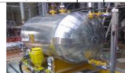
PROJECT PD2 REHABILITATION - Installation of Calcium Silicate for Vessel Drum at Tungku Jaafar Power Plant Port Dickson, Negeri Sembilan
